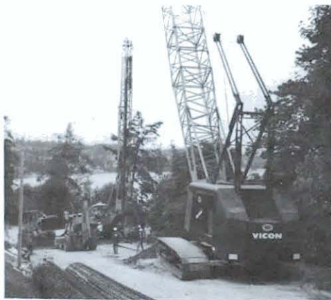
The project includes the drilling of piles.
